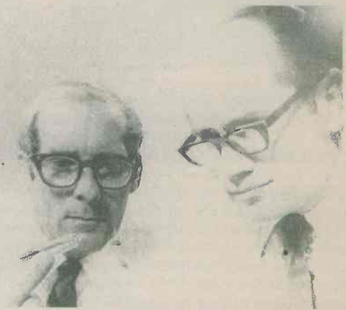
Here, Albert A. Ballam holds a lithium tantalate crystal with David W. Rudd looking on. Lithium tantalate crystals have Q factors which enable them to supersede traditional quartz crystal units
